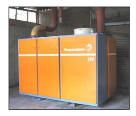
With an eye on productivity and the other on long term investments to achieve top company performance over the next decades, MIDDLE EAST GLASS in Egypt updated the vacuum system to serve the IS machines supplied by EMHART first in 2004 with one UV50 pump and again in 2005 with the second unit UV50.
