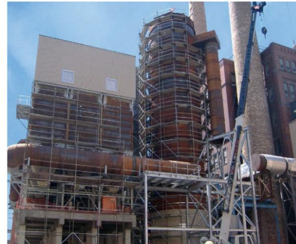
Once the modules, hoppers, scrubbing tower, and manifolds have been erected, insulation is applied prior to the installation of the exterior siding.
