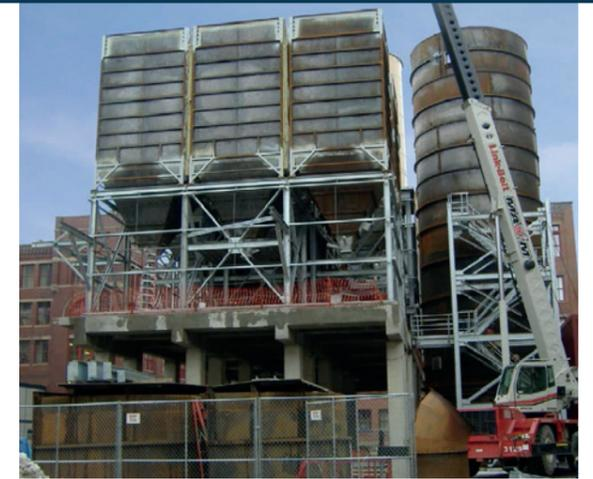
With the foundation work completed, and the structural steel erected, the last of the modules for this catalytic filter system is lifted into place.
