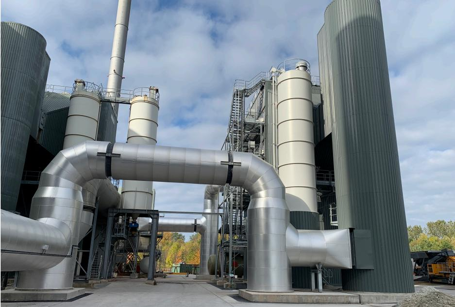
Because of regulatory requirements in summer 2006 Interprojekt added a SCR reactor with catalysts and ammonia water storing and dosing system to the existing installation.
