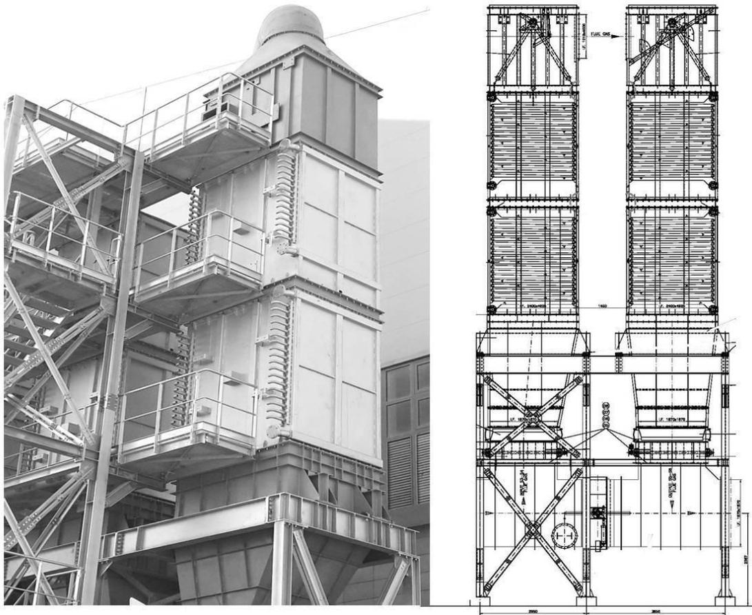
ORC used belong to the last generation. It uses a combined radial or radial-axial high efficiency turbine. The organic fluid used is cyclopentane, having thermodynamic properties optimal to achieve the best efficiencies using thermal oil in the range of 300°C. This fluid also allows a direct condensation in air cooled condensers, being the best choice for the plant location; actually in this specific place water is only partially available and ambient temperatures are typically continental.
